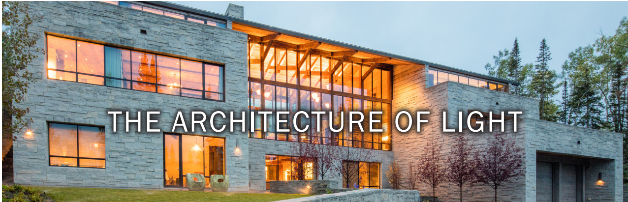
Mountain Village Residence, Lighting Design by Robert Singer & Associates
